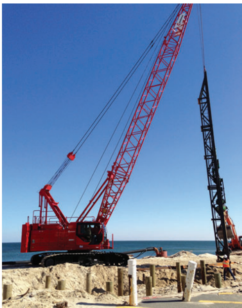
Albert Marine Construction used an 80 tonne capacity Manitowoc 8500-1 for clean-up work in the wake of Hurricane Sandy. The crawler crane was used for piling work to rebuild the mile-long (1.6 km) Lavallette Boardwalk on the Jersey Shore.
