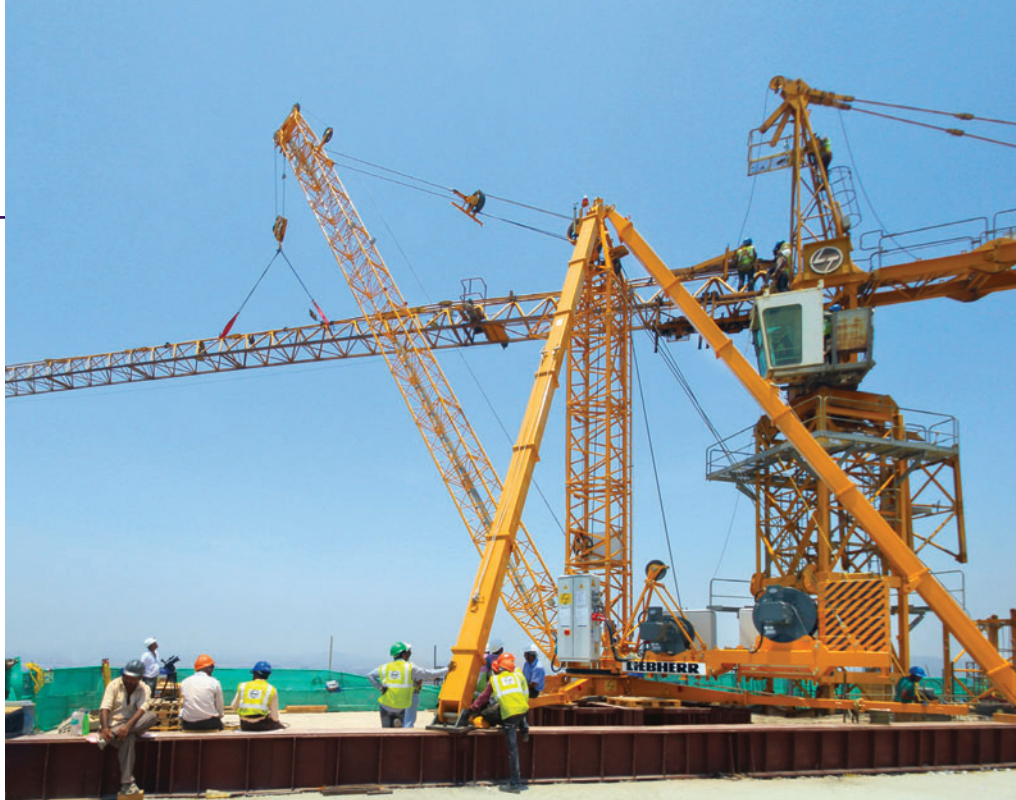
Contractor Larsen & Toubro used a Liebherr 200 DR 5/10 Litronic Derrick crane to dismantle a tower crane on the 220 m Kohinoor Tower in Mumbai, India.
